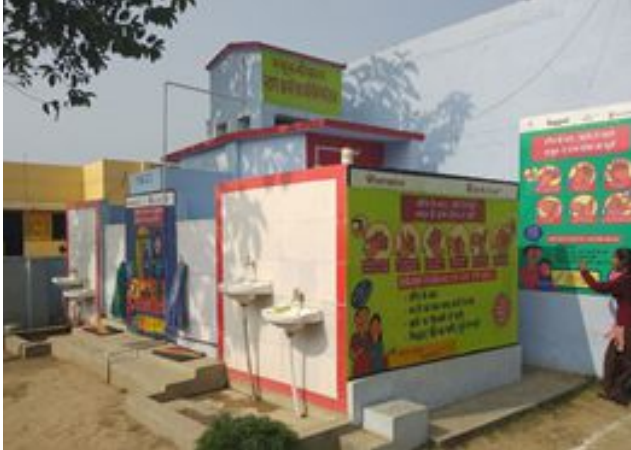
School Sanitary Block of UPS, Kauwapur
