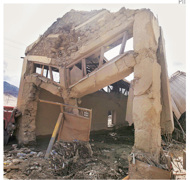
A building in Choglumsar near Leh that was
